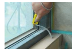
Pull the remover backward to peel the silicone.
