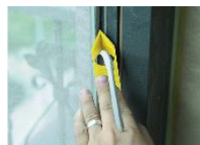
Push the remover backward to scrape the silicone.
